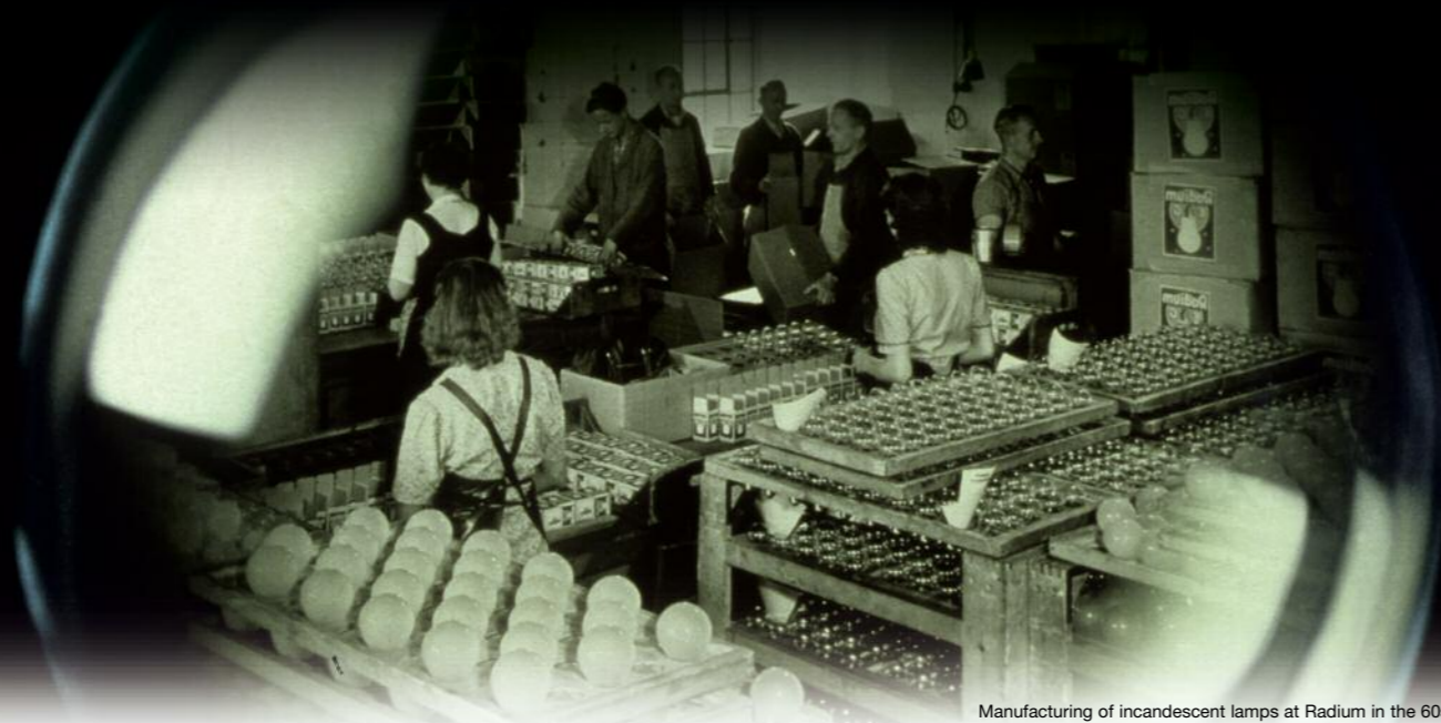
Manufacturing of incandescent lamps at Radium in the 60s
